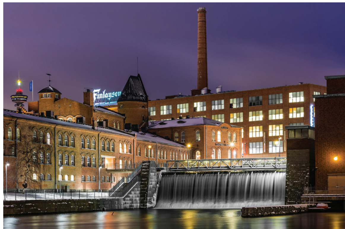
A dam over the Tammerkoski rapids in the Finlayson industrial area of Tampere.
